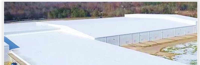
Rome, GA, USA: US Distribution Centre Surface: 30.660 m 2
