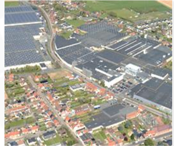
Sint-Baafs-Vijve, Belgium: Head Office, Showroom, and Production Surface area: 306.000 m
