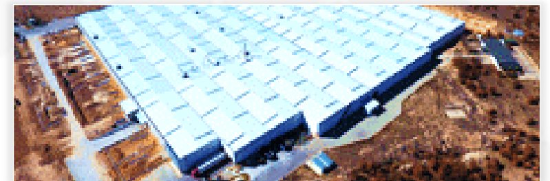
Usak, Turkey: Production Surface: 273.000 m 2 , 86.520 m 2 (covered area)
